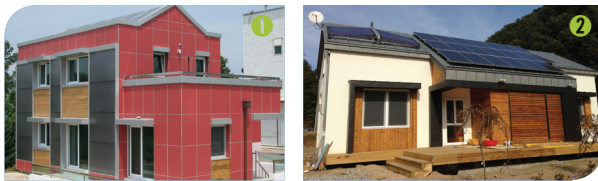
[Fig 1] Vertically-installed facade-integrated flat-plate solar collectors
